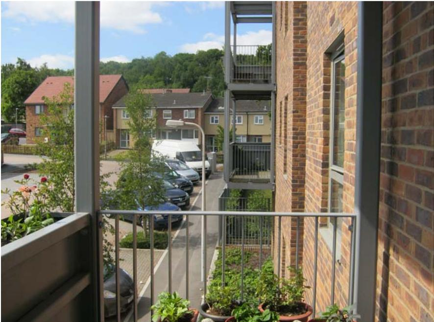
**Figure 9: Corridors with large opening windows provide cross-ventilation throughout communal spaces (as well as for flats/bedrooms)**
