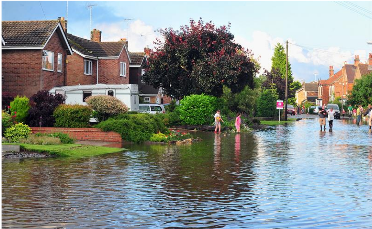
Flooding in Rolleston on Dove, Staffordshire in 2012. Image courtesy of Rolleston on Dove village website
